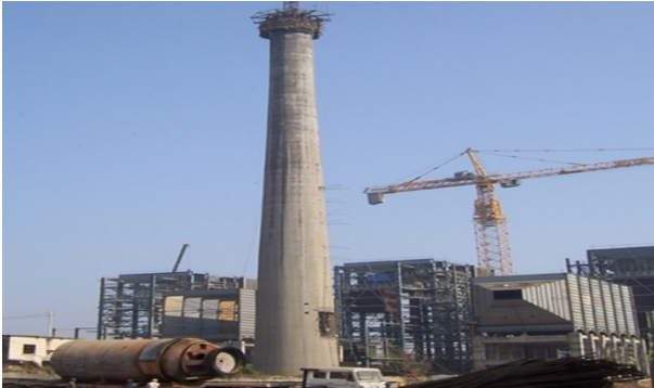
Fig. 1 Insights of RC Chimney
